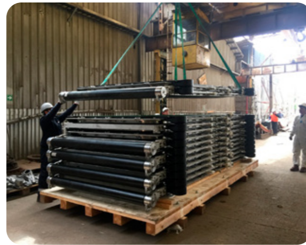
Complete plate pack installation
