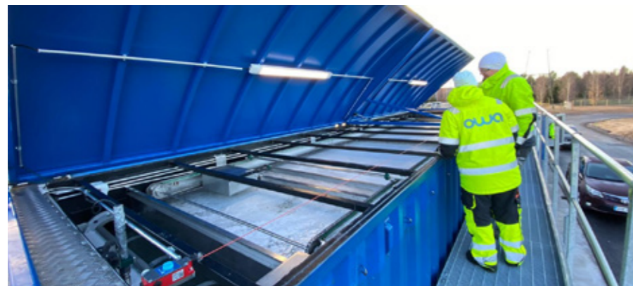
We understand the wastewater treatment is not your core business. That is why we also offer setting up the wastewater treatment processes.
